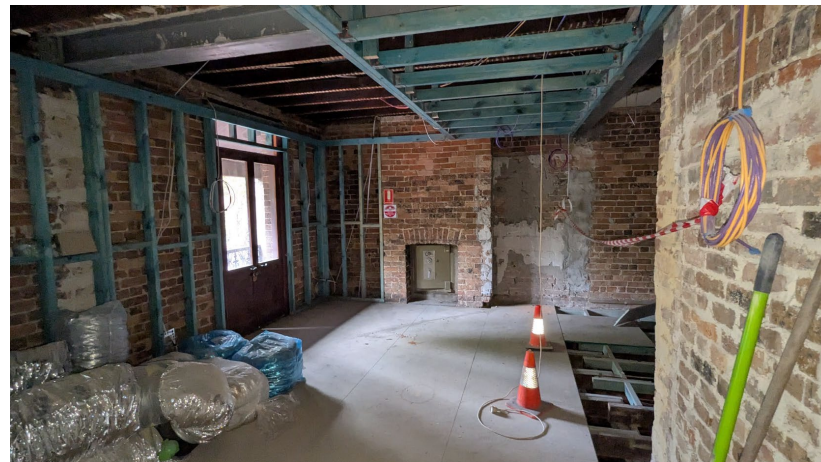
Internal building condition
