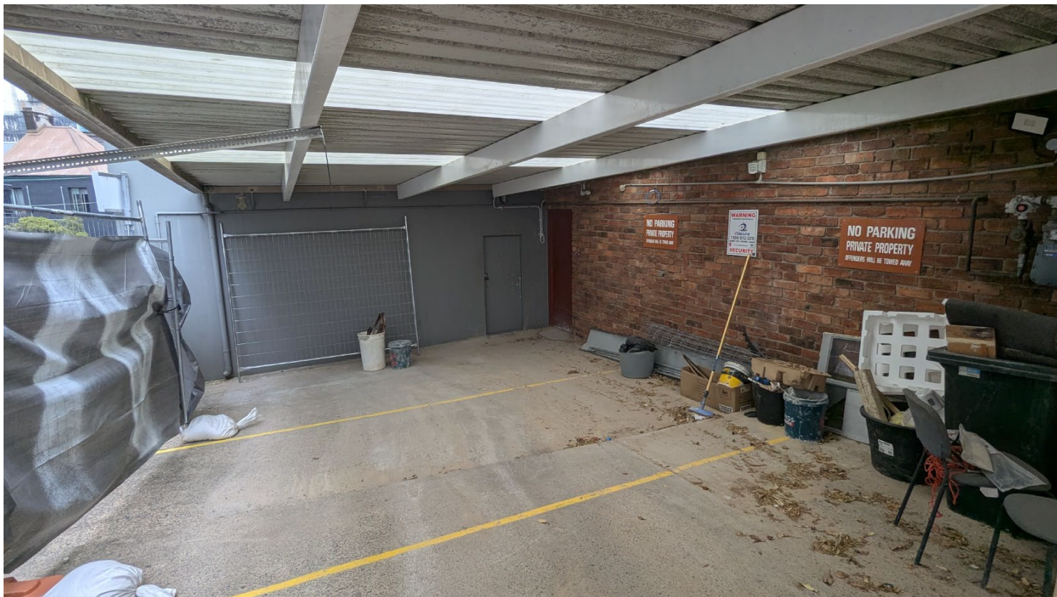
Existing covered hardstand parking area at rear
